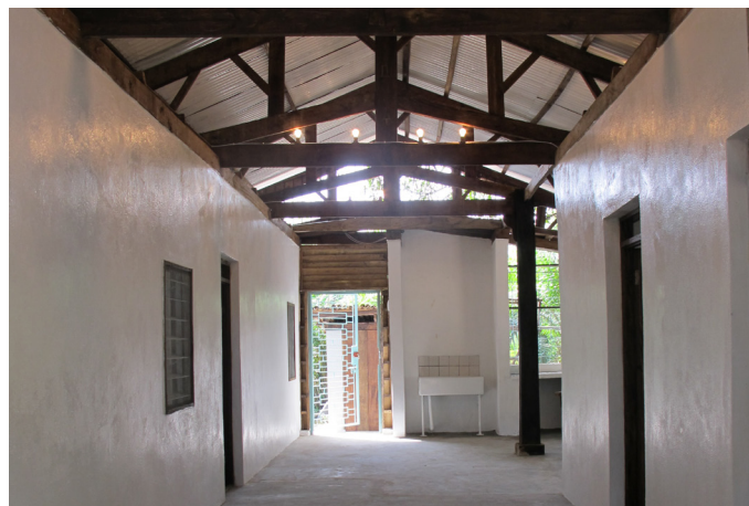
Fordelingsgang i Paulas House
